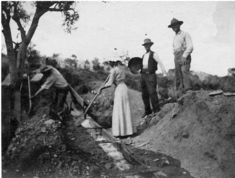
Ines Fraser adds promising soil to the gold-separation sluice at the Los Alamos mine. (Courtesy of Connie Fraser Kiely, circa 1910)
