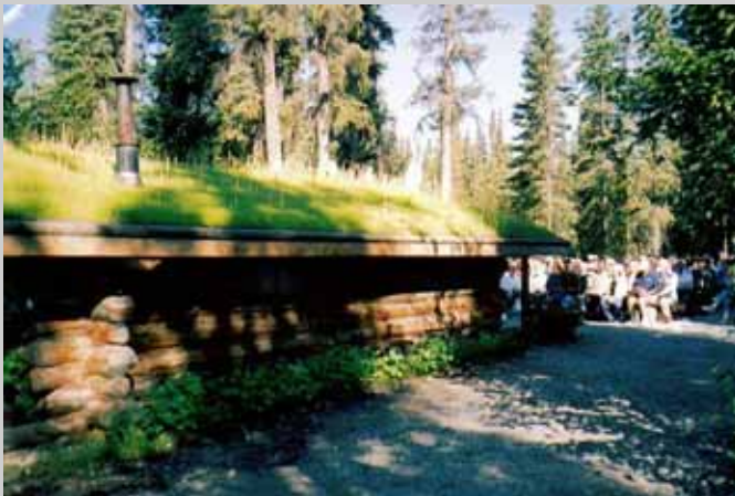
Sod roof... needs cutting!!
